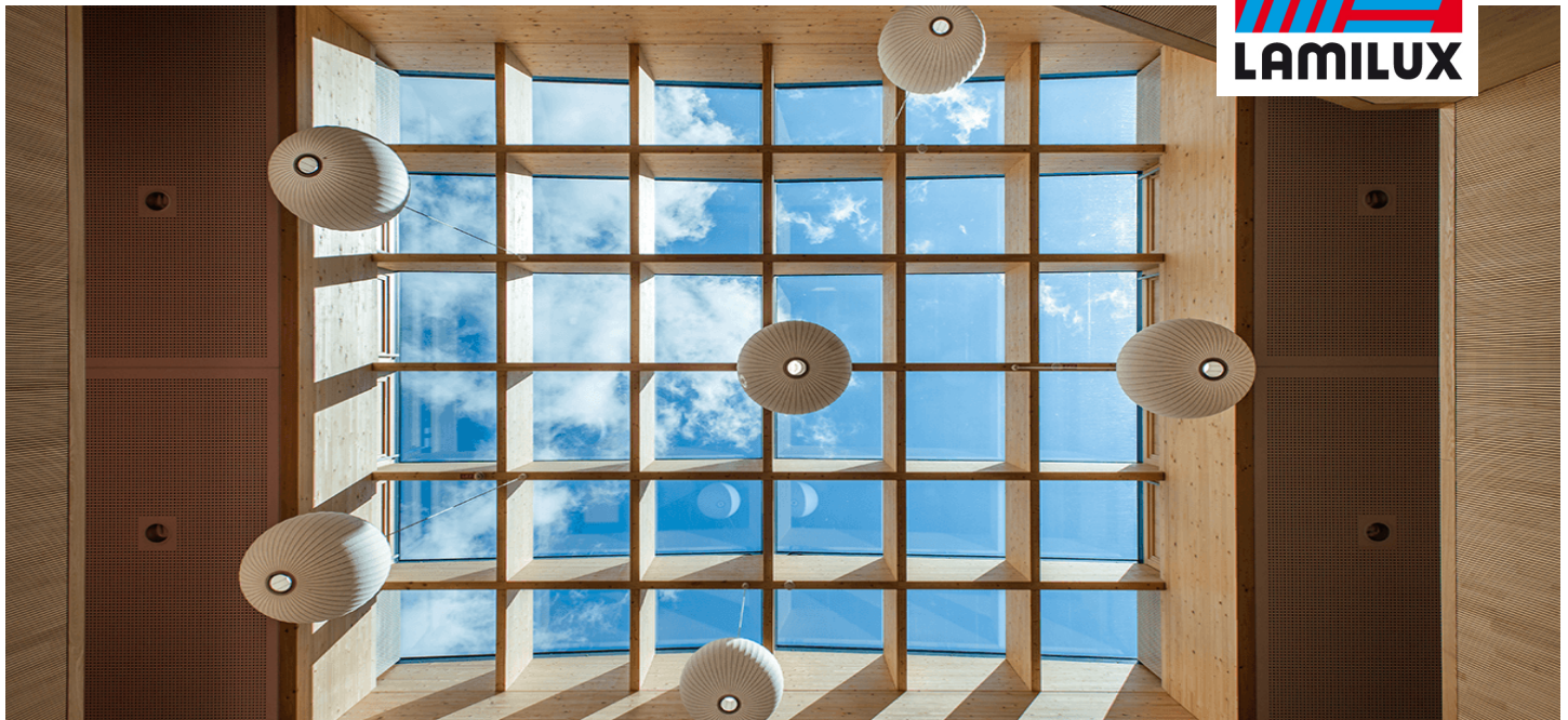
Day Care Centre, Frankfurt
